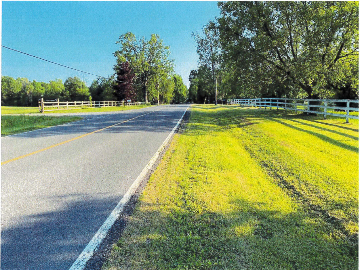
Figure 9: Looking South from the Proposed Site Access
