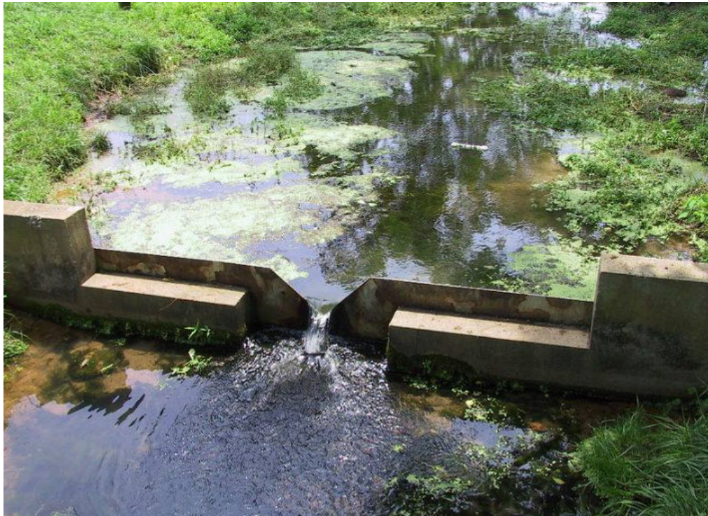
Figure 5-1: V-notch Cast-In-place Concrete Weir Wall Illustration
