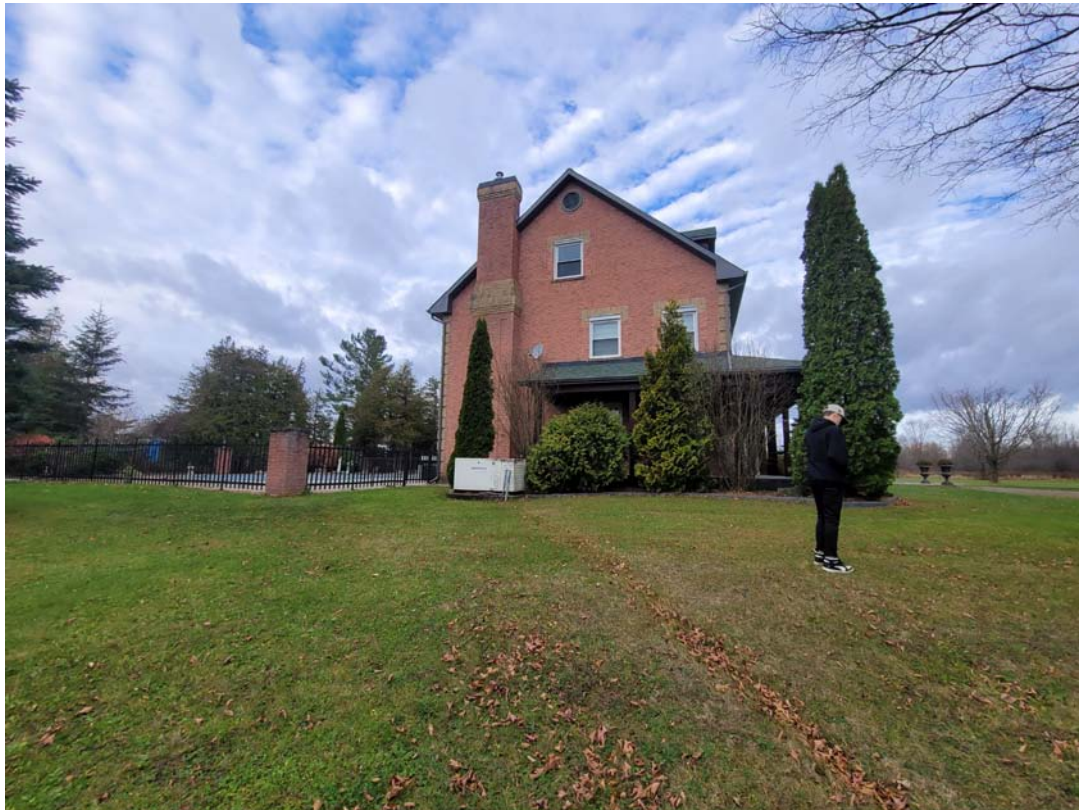
South side view of single family dwelling
