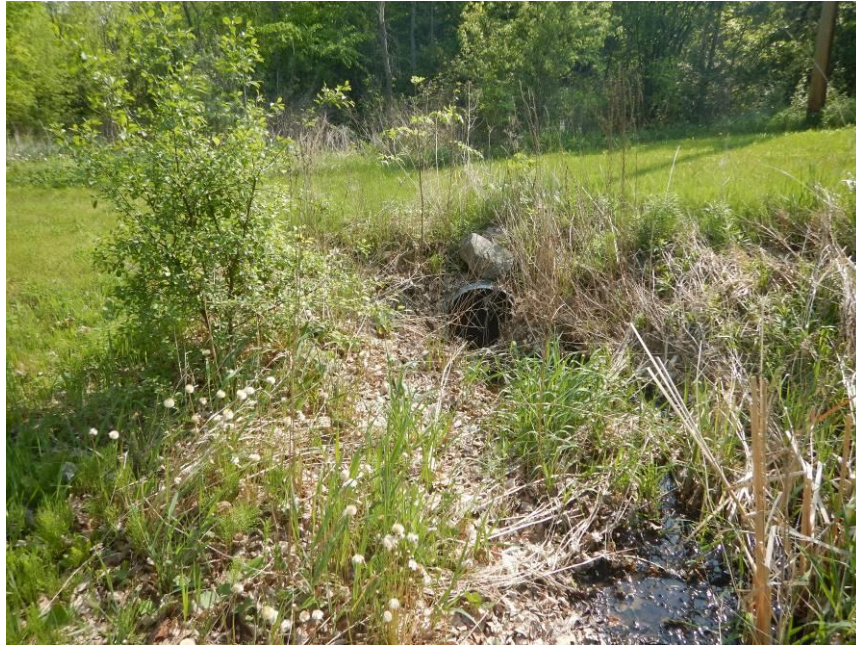
Photo 15: Tributary 2 looking at the upstream end with the crossing (May 21, 2022)
